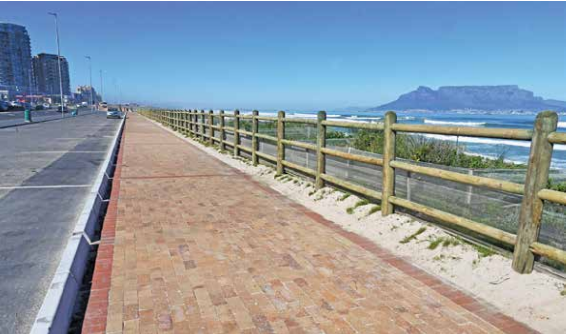
Way better walkway: The upgrade at Table View beachfront includes a supersized walkway, some 4 m wide and 2 km long.
