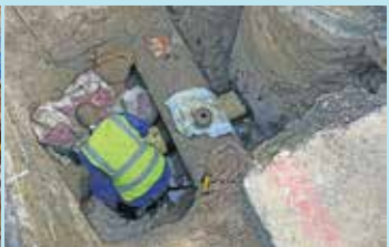
Dig-and-CIPP combo: For the rehabilitation of sewer pipes in Century City, completed late last year, the City used a combination of open-trench repairs and cured-in-place pipe (CIPP) lining.
