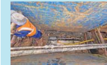
Dig-and-CIPP combo: For the rehabilitation of sewer pipes in Century City, completed late last year, the City used a combination of open-trench repairs and cured-in-place pipe (CIPP) lining.
